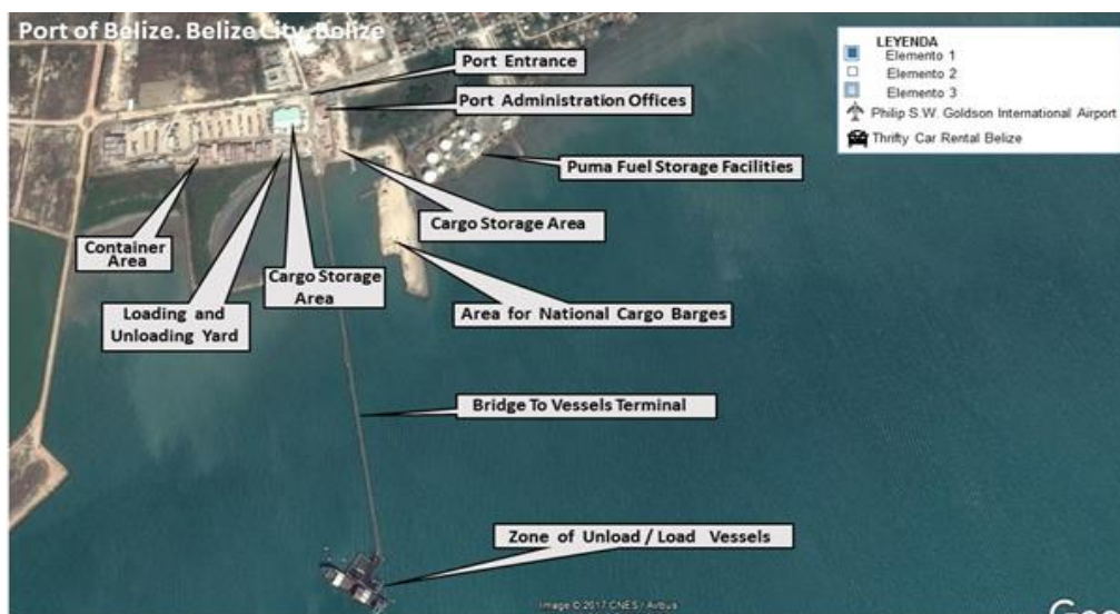
Figure 2: Port of Belize Harbour (Source: Schweikert and Ashcroft, 2017)
